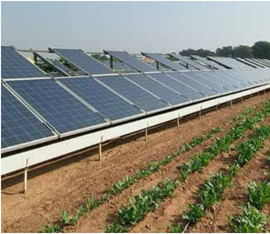
FIGURE 6.2 105 kW APV at ICAR-CAZRI, Jodhpur, Rajasthan
